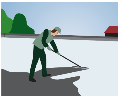
Manual Roof coating application
