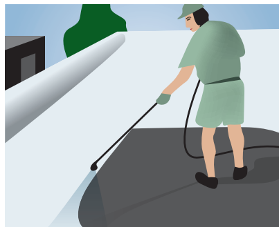
Roof coating with airless spray equipment
