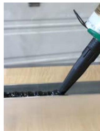
Figure 16: Applying the silicone sealant for weatherproofing
