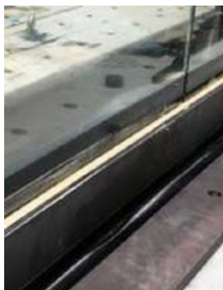
Figure 14: DOWSIL™ 375 Construction & Glass Embedding in U-profile
